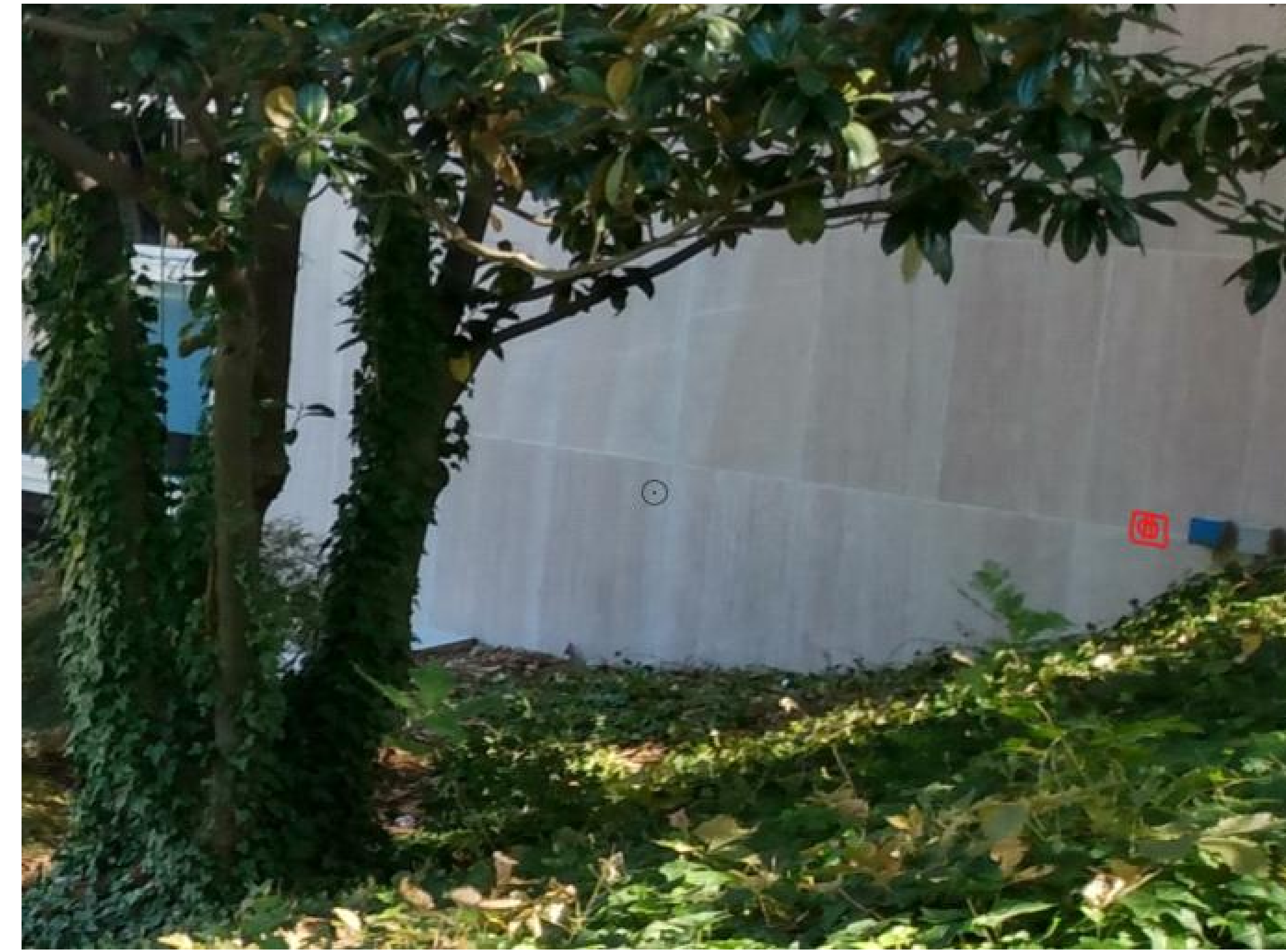
2 WEST - DRAINAGE IMPROVEMENTS - PHOTO #1
