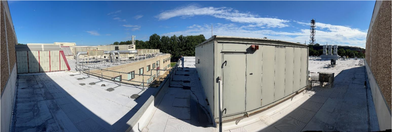
Photo #22: Connection between Mechanical Building and Roof D
