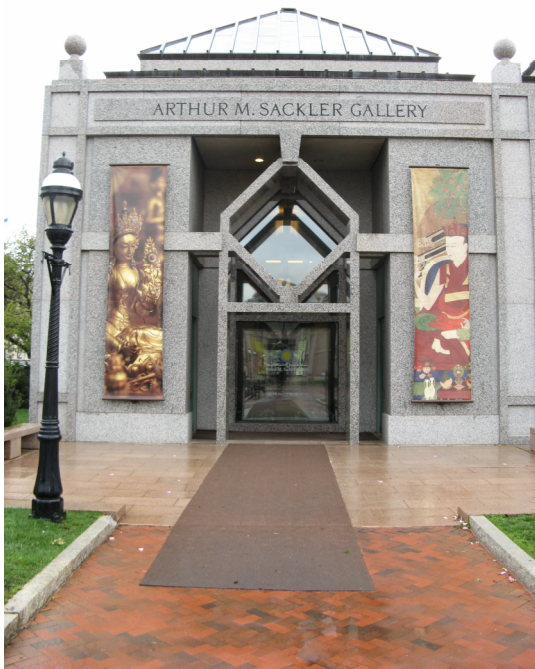
Photo 02 Main entrance from Haupt Garden.
