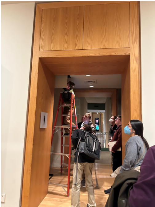
Photo 13: Corridor to Men's room. Ceiling is wood and GWB. Piping may cross above to Men's room.
