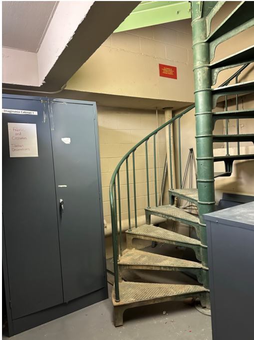
Photo 10: spiral stair to Mezzanine 0014. Mezzanine 0014 is above the Level B1 toilet rooms. Space will be sprinklered.
