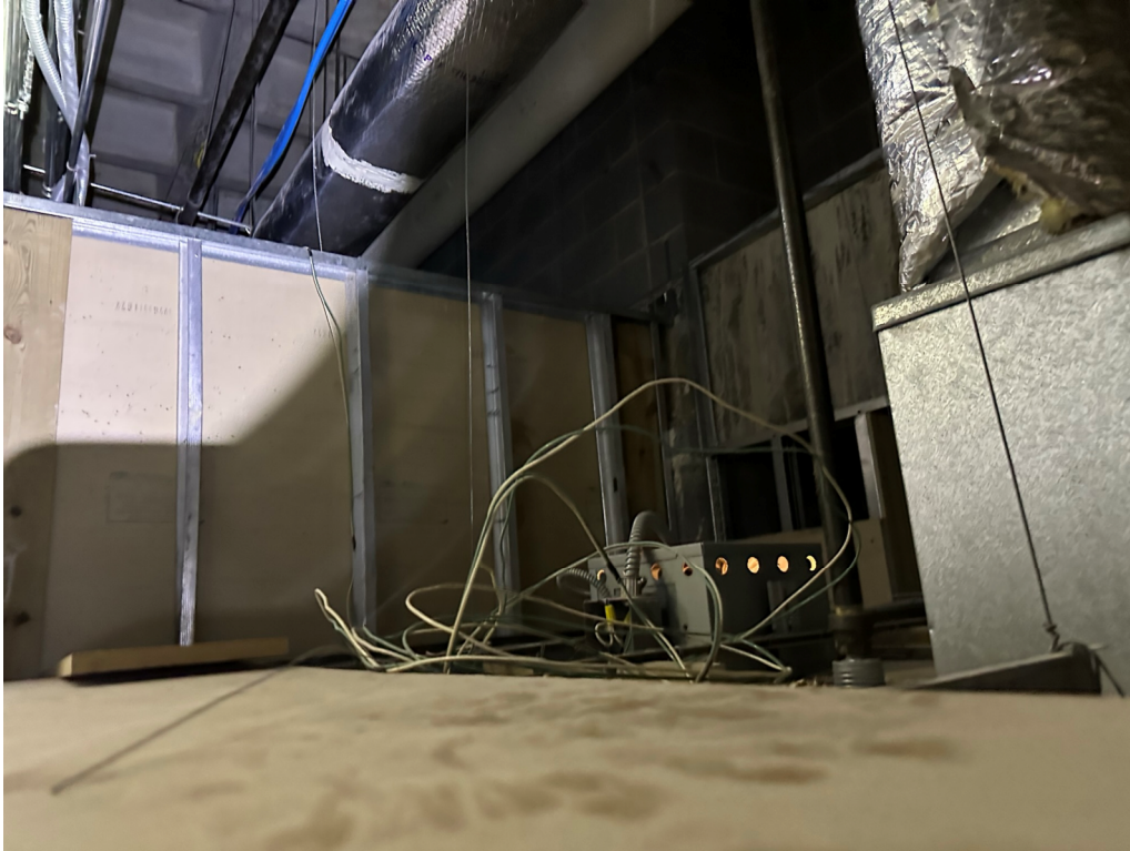
Photo 14: Above ceiling to Men's room,
