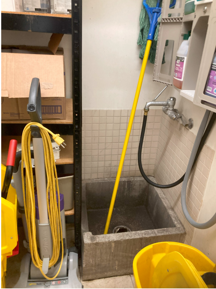
Photo 18: Janitor's Closet 3023. This room will include a 36 x 36" slab removal to access to a sanitary line below the slab.
