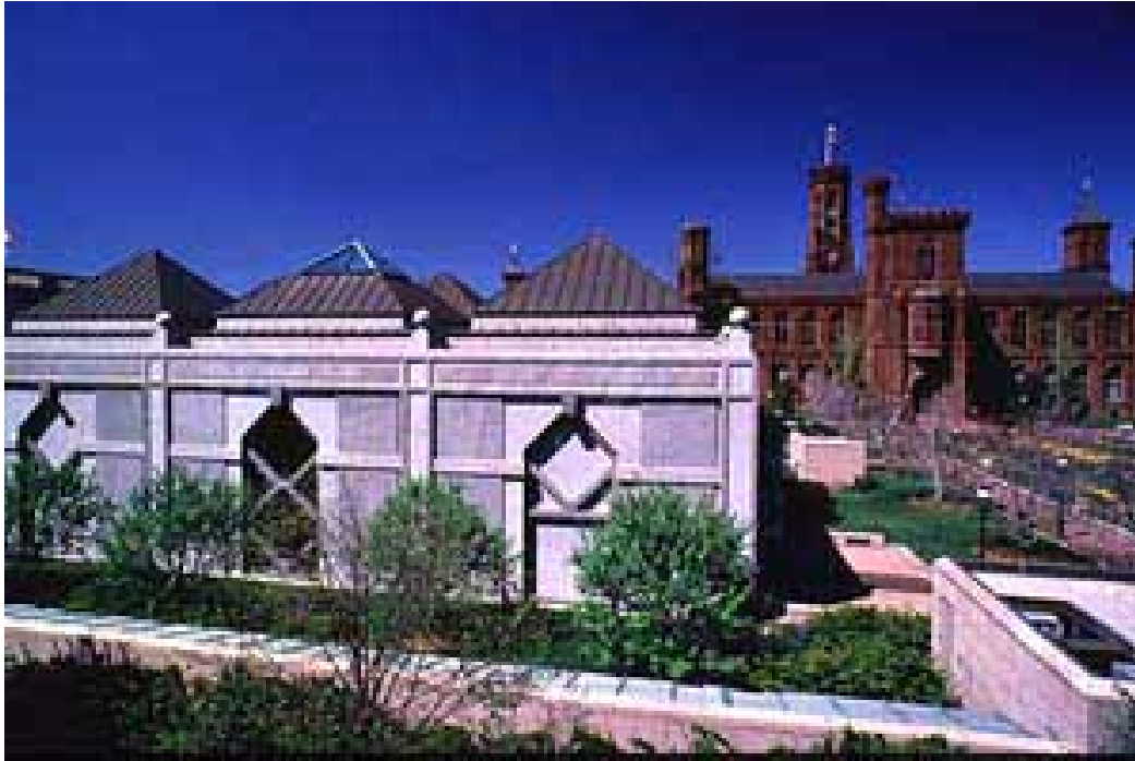
Photo 01: Sackler Gallery Pavilion. SW corner of Quadrangle Building
