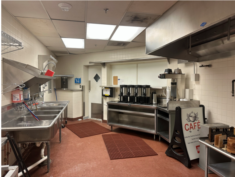
Photo 16: Kitchen 2020: ETR 3-compartment sink; range has been removed and gas capped; see new layout for new equipment.
