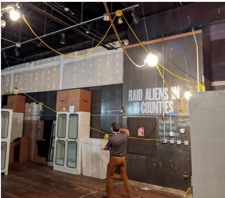
Figure 09: Inside AMPU Storage, looking towards security wall with expanded mesh.
