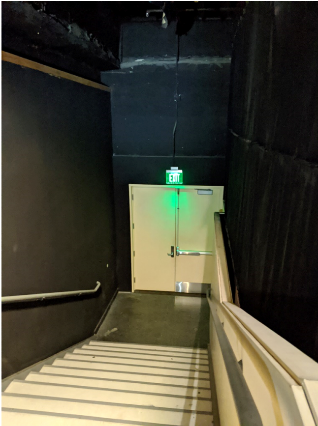
Figure 08: Stair from upper mezzanine to be demolished. Door to American Presidency is ETR but a delayed egress function will be added.
