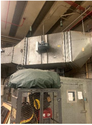
EF-7 – Serves the spraybooth in the African Art paint shop. Starter location 1118ER / Breaker Panel HDP1B.
