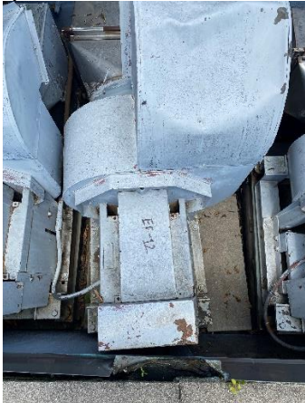
EF-12 – Serves room 1115 fume snorkel. Located on the rooftop of stairwell 1006. Switch operated in the space. Starter location 1118ER / Breaker Panel LP1B1 #2.
